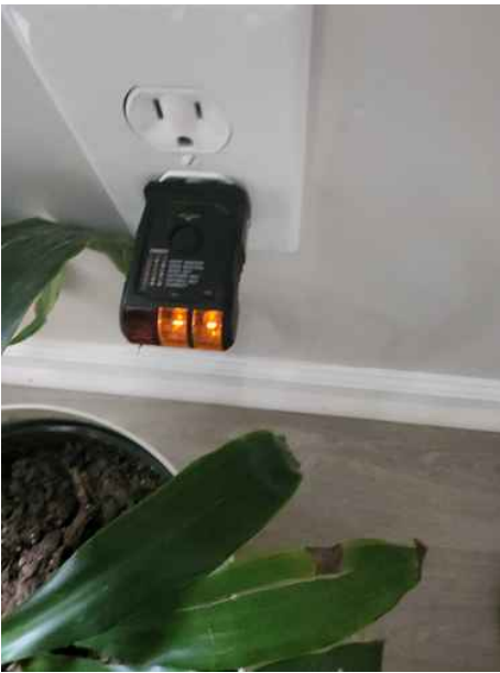
LIGHTING Satisfactory Notes:
